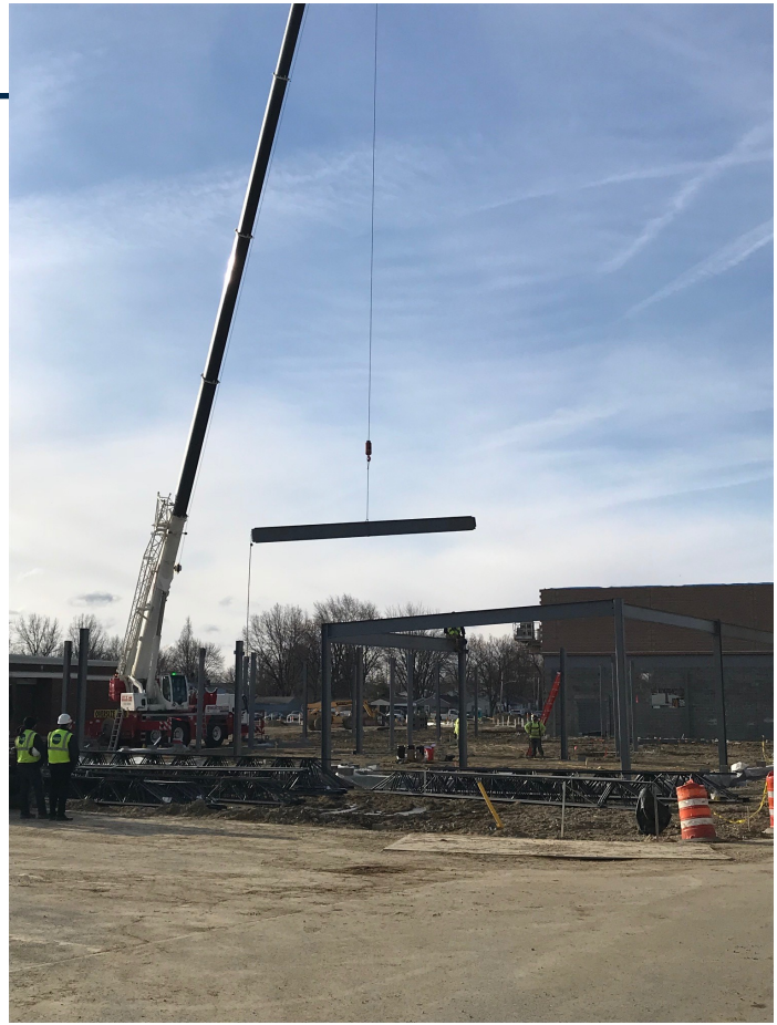
LONGFELLOW STEEL BEAMS
