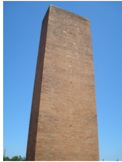
Large chimney at east end of 1955 Original Construction
