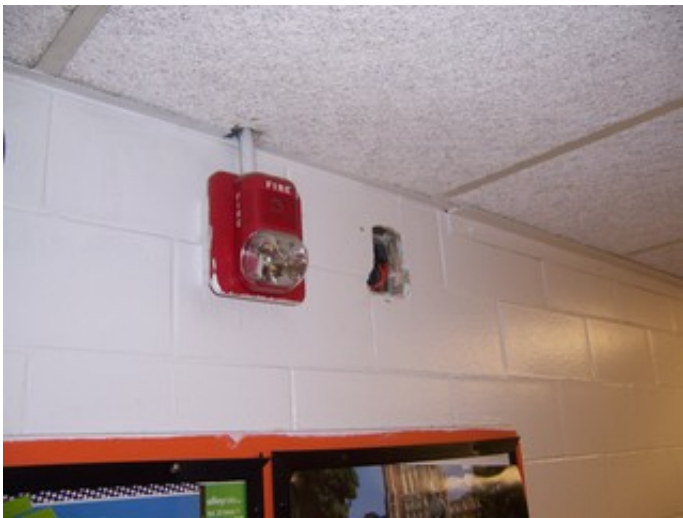
Wall Mounted Fire Alarm Strobe
