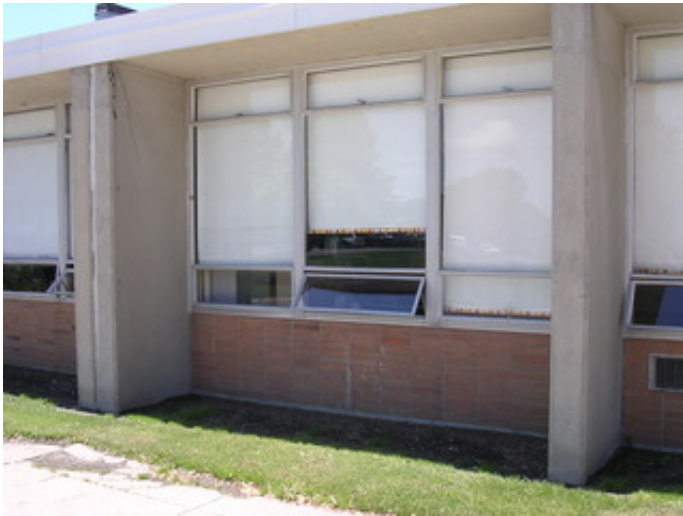
Typical aluminum windows.
