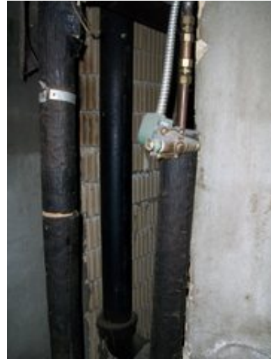
Sanitary drainage Piping
