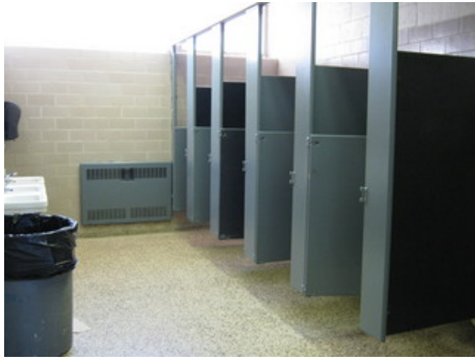
Non accessible group toilet room
