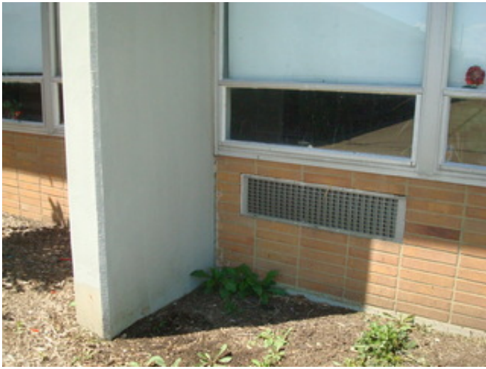
Exterior piers on 1955 Original Construction
