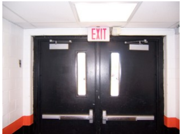
Ceiling Mounted Exit Sign
