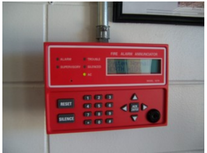
Fire Alarm Control Device
