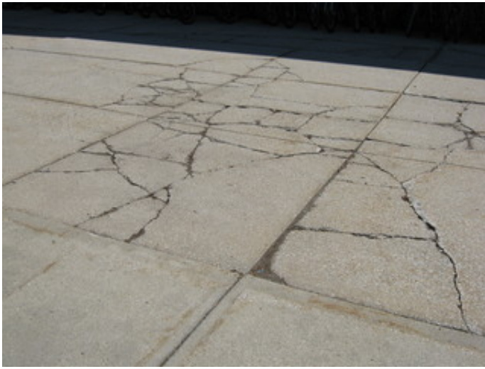
Sidewalk in poor condition
