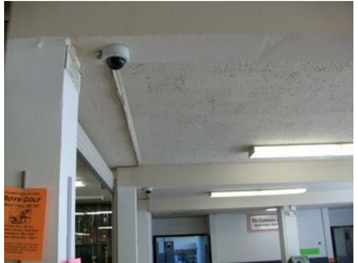
Ceiling Mounted Surveillance Camera
