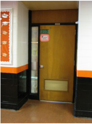
Typical recessed classroom door
