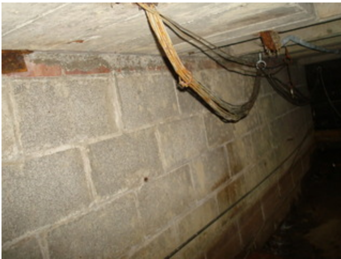
Crawl foundation wall
