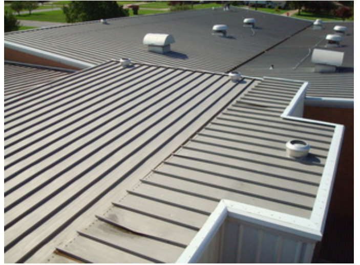
Metal roofing retrofit surfaces on the 1955 Original Construction
