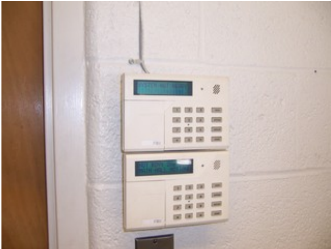
Security Alarm Panels
