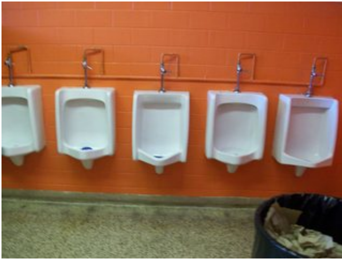
Toilet room fixtures
