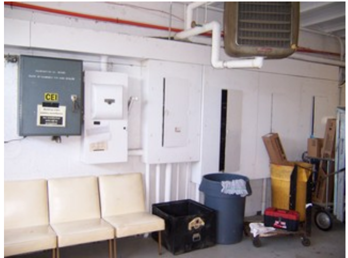
Main Electrical Switch and Panels
