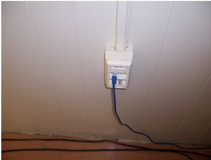
Classroom Technology Outlet
