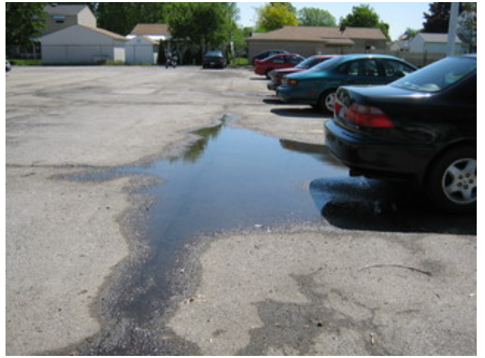
Parking lot ponding
