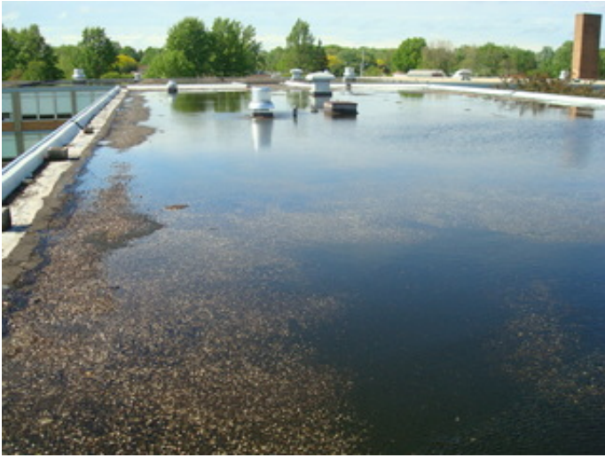
Standing water on 1962 Addition
