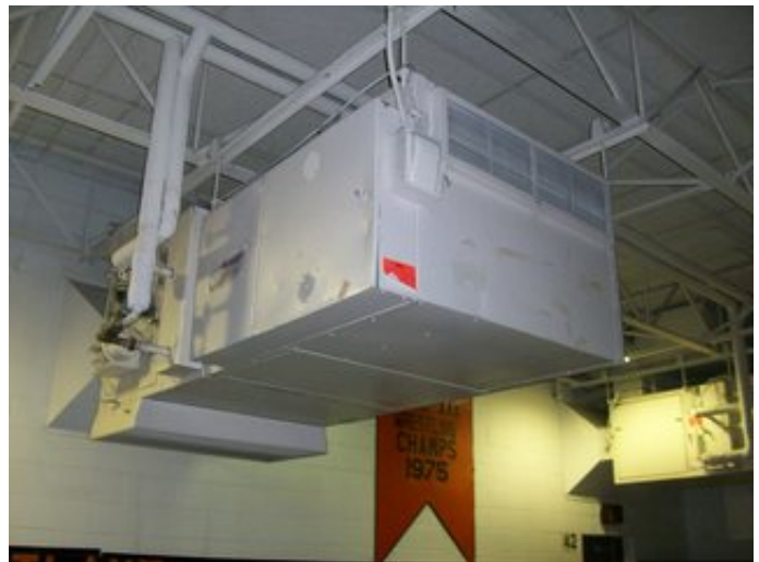
Forced Air Heating Unit
