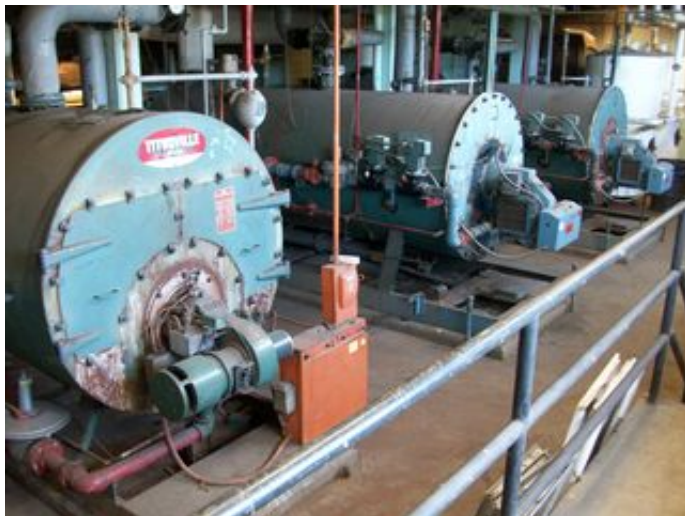
Gas Fire Hot Water Boilers
