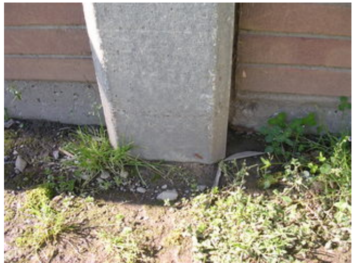
Typical foundation condition.
