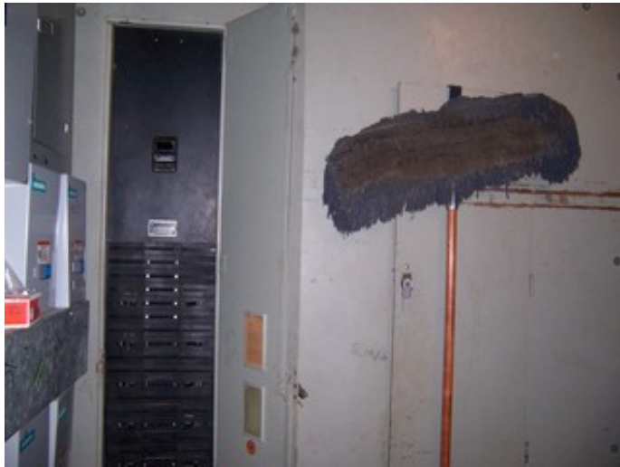
Secondary Electrical Panels
