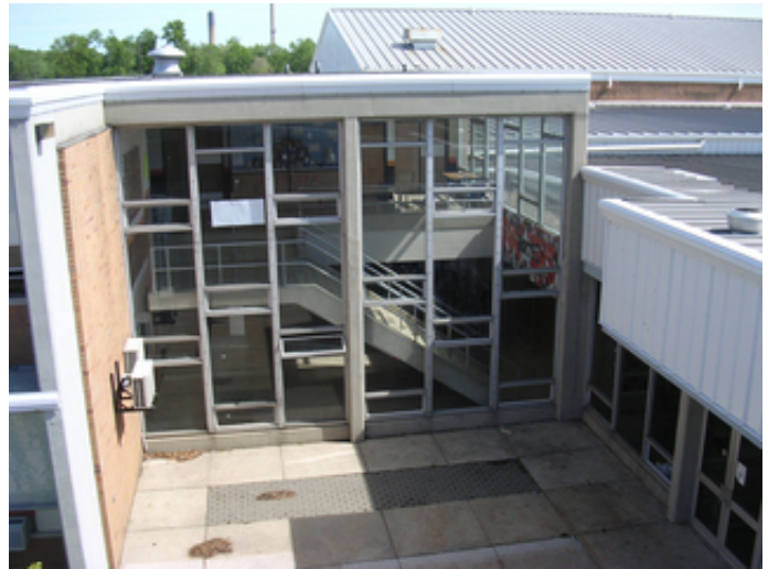
Typical aluminum curtain wall system.
