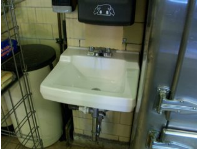
Sanitary drain below sink
