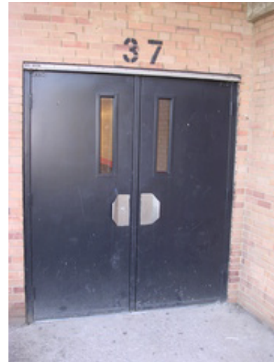
Typical hollow metal doors.
