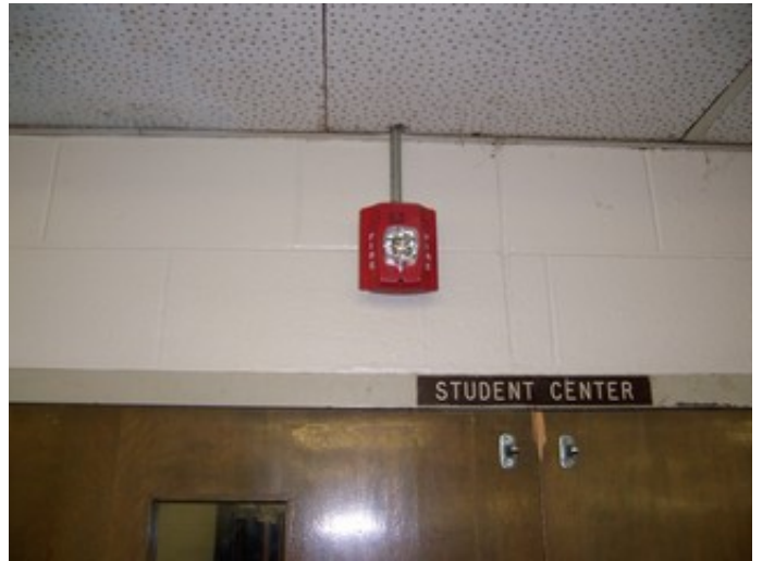
Fire Alarm Strobe
