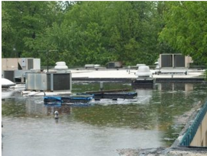
Roof Top A/C And Exhaust Fans
