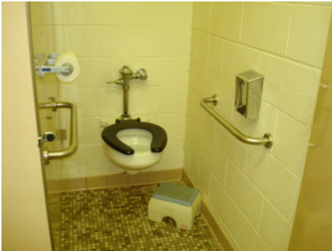
Toilet with grab bars
