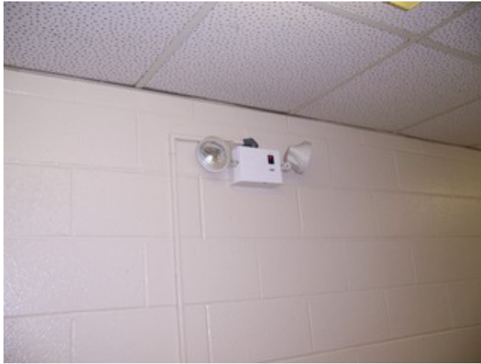
Wall Mounted Emergency Lighting
