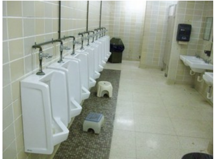
Domestic water piping at plumbing fixtures
