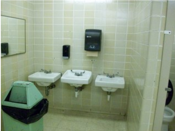
Sanitary drain below sink
