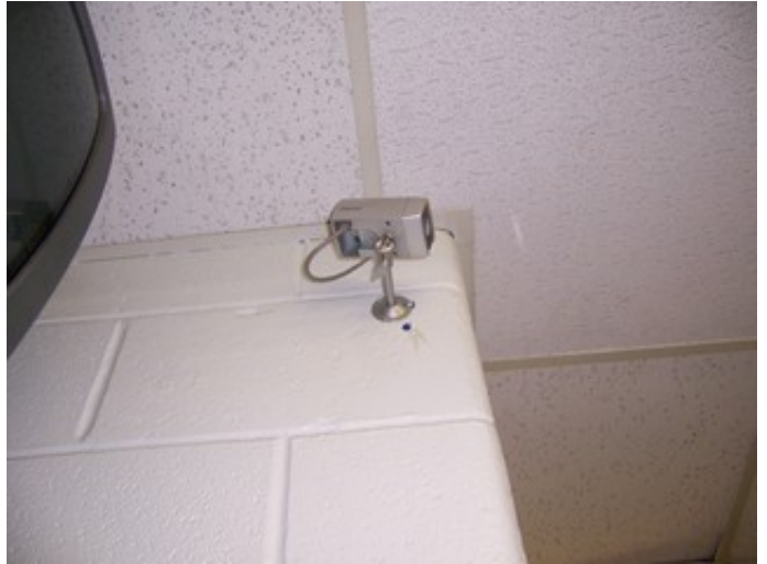
Wall Mounted Security Camera
