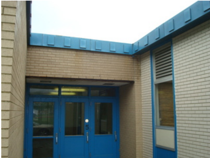
Rusted lintel and deteriorated control joint in 1970 Addition
