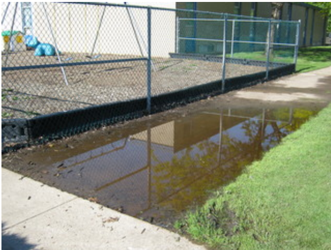
Sidewalk ponding
