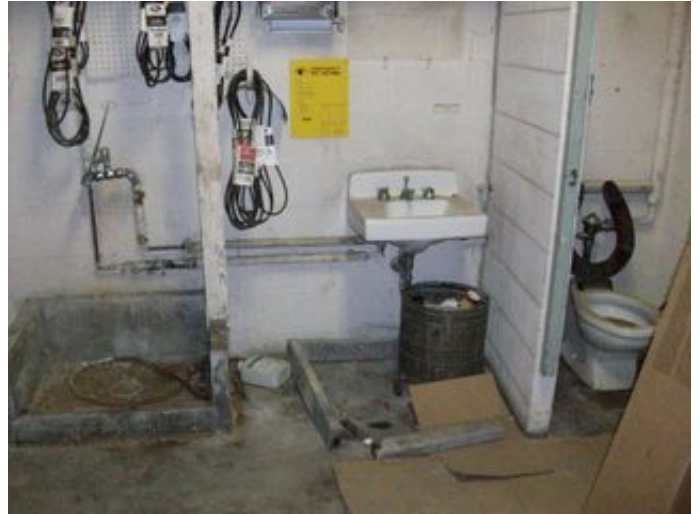
Sanitary drain below sink
