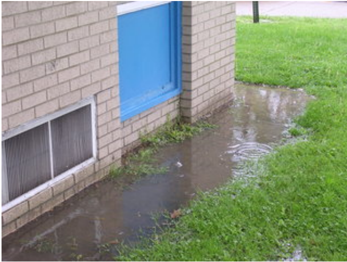
Ponding at foundation.
