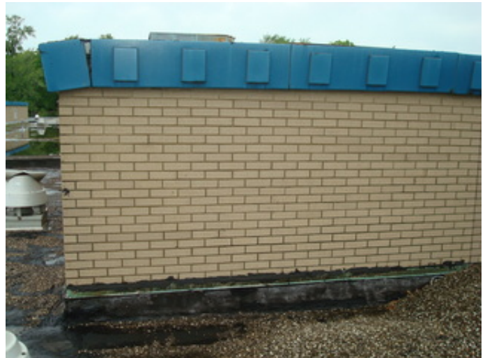
Deteriorated metal wall coping
