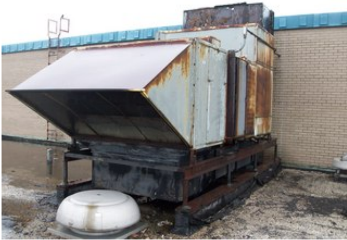
Air Handler With Electrical Heating Strips
