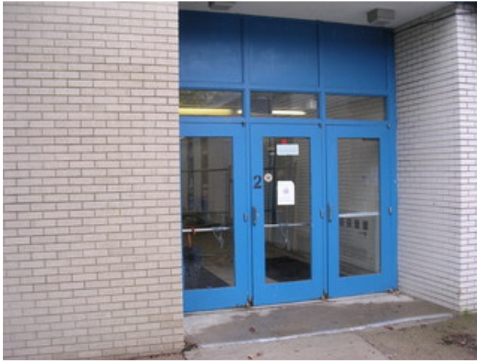
Typical hollow metal glazed doors.
