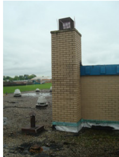
Chimney showing deteriorated mortar
