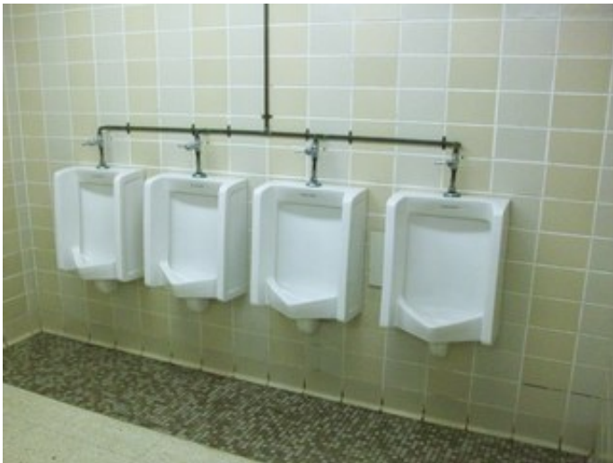
Toilet room fixtures
