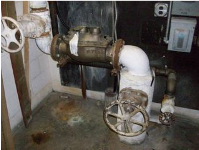
Domestic Water Piping
