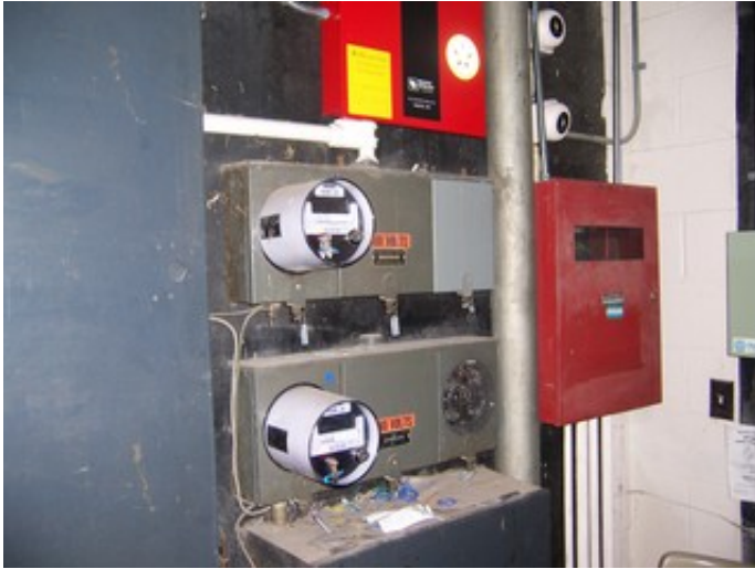
Electric Utility Meters
