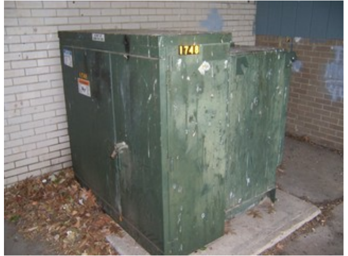
Pad Mounted Transformer
