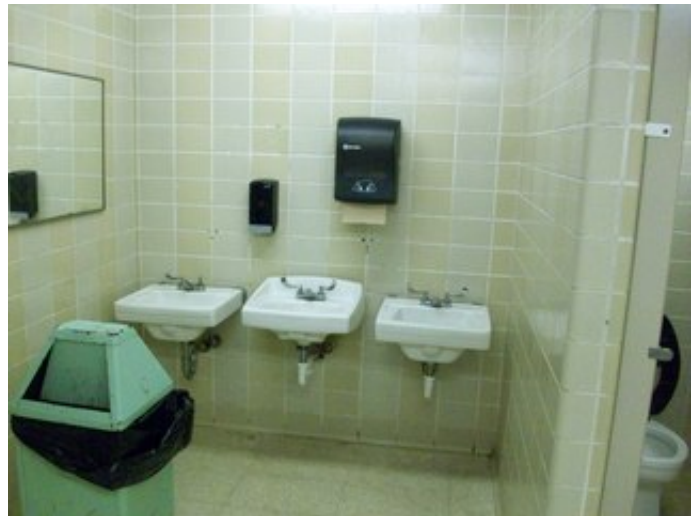
Toilet room fixtures
