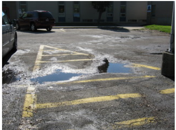
Parking lot ponding
