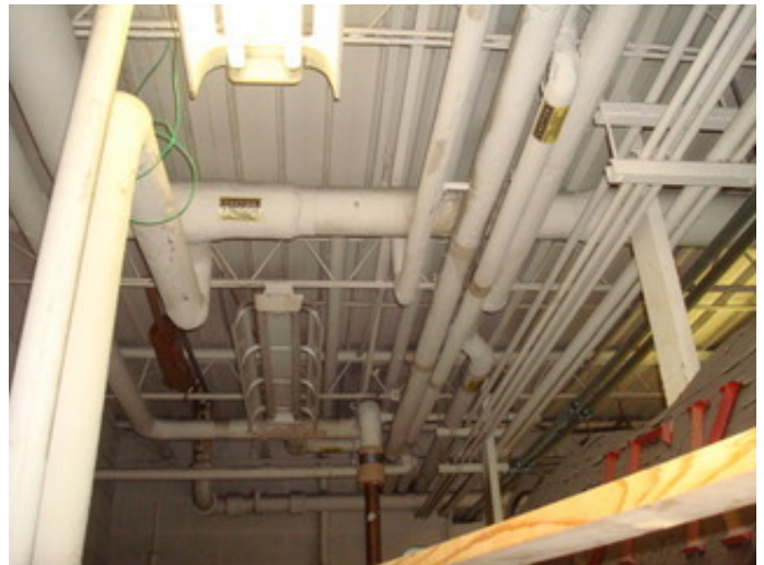
Pipe insulation
