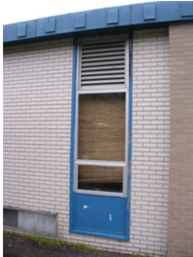
Typical aluminum window in hollow metal frame.
