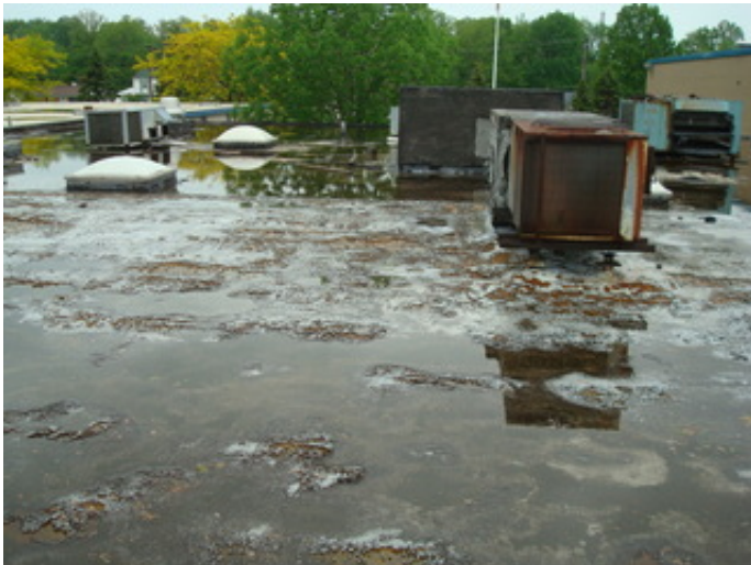
Spray-on roofing, standing water, and skylights
