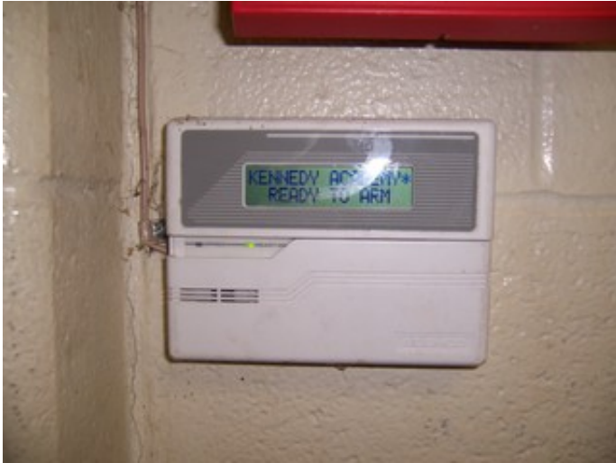
Security Alarm Panel
