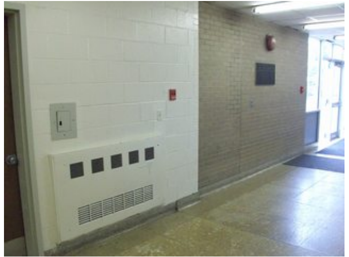
Electric Unit Heater
