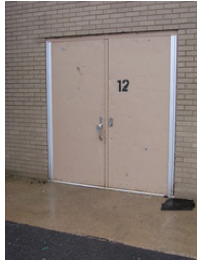
Typical hollow metal doors.
