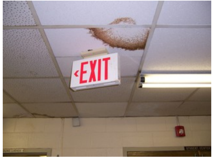
Ceiling Mounted Exit Sign
