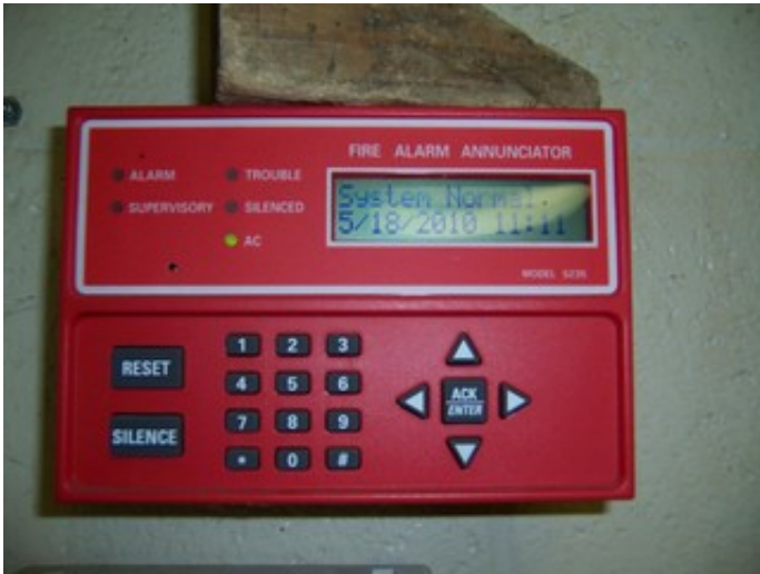
Fire Alarm Control Device
