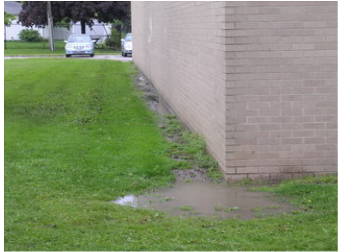
Ponding at foundation.
