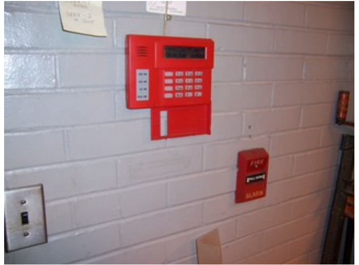
Fire Alarm Devices
