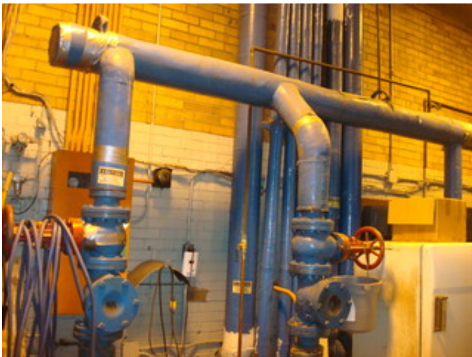
Pipe insulation and fittings
