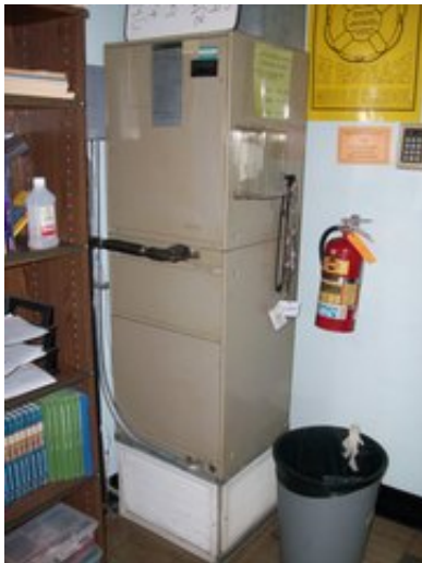
Computer Room Split A/C Unit
