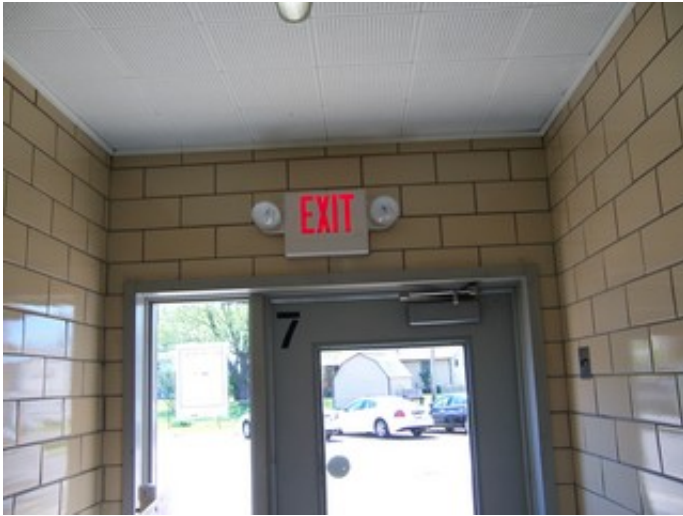
Typical Exit Sign
