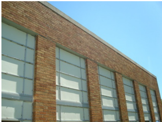
Rusted lintels and damaged brick in 1949 Original Construction
