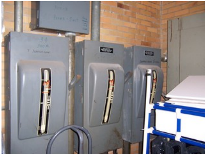
Campus Main Disc. Switches
