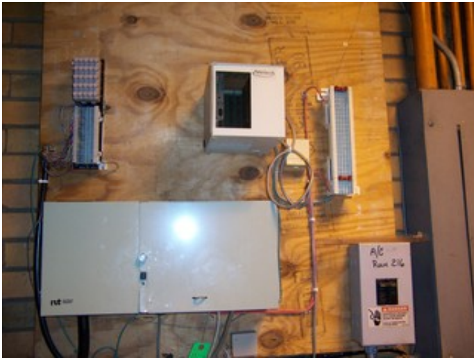
Security Headend Equipment
