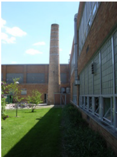
Chimney is in poor condition.
