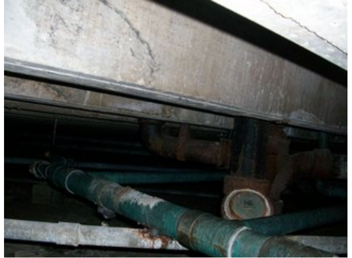
Sanitary drainage Piping
