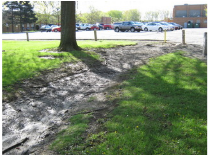
Evidence of erosion
