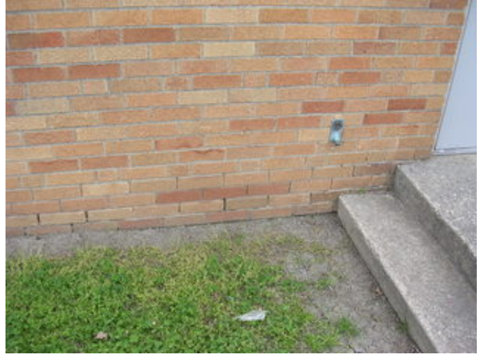
Typical foundation condition.
