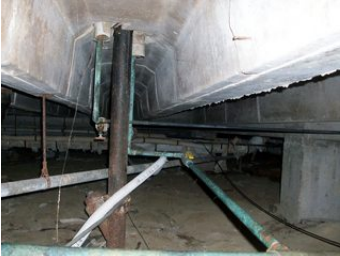
Sanitary drainage Piping
