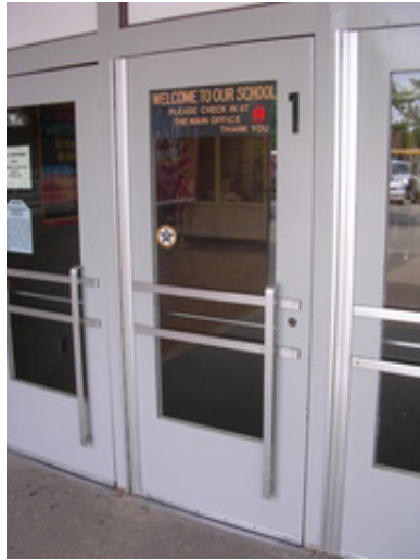
Typical entry door.
