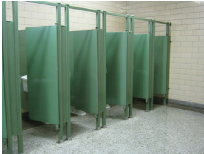
Non-compliant toilet partitions
