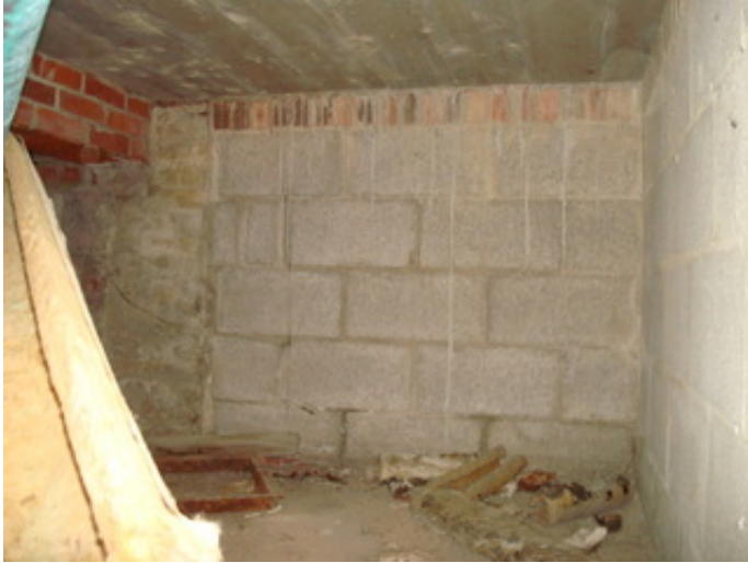
Crawl space wall.
