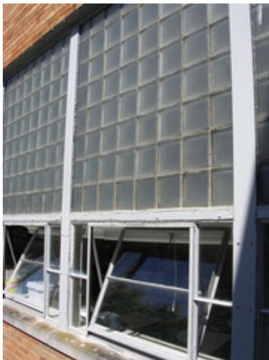
Typical window w/ glass block.
