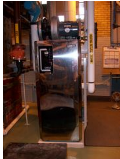
New High Efficiency Hot Water Boiler
