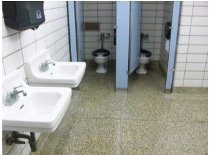
Toilet room fixtures
