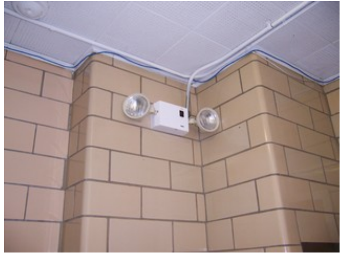
Typical Emergency Light
