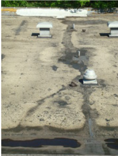
Ponding, patches and damaged roof drains on 1957 Addition
