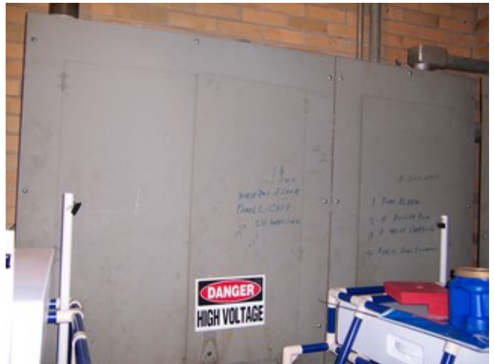
Main Distribution Switchboard
