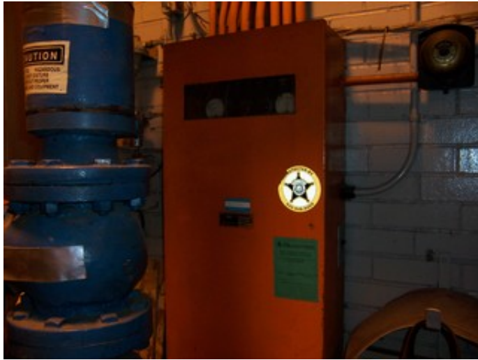
Fire Alarm Control Panel
