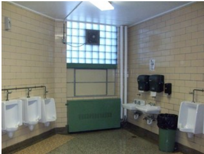
Toilet room fixtures
