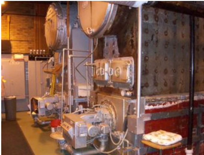
Original Gas Fired Hot Water Boilers
