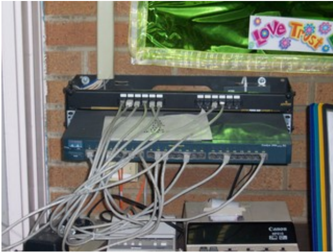
Technology Head-End Equipment Rack
