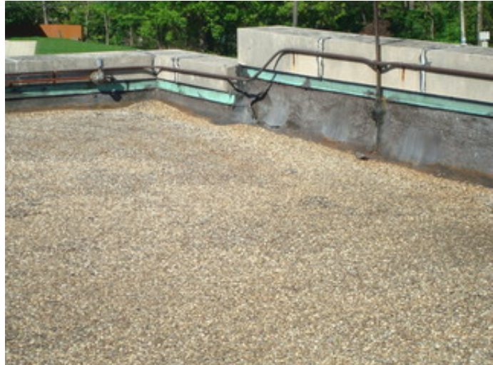
Damaged wall flashing on 1949 Original Construction
