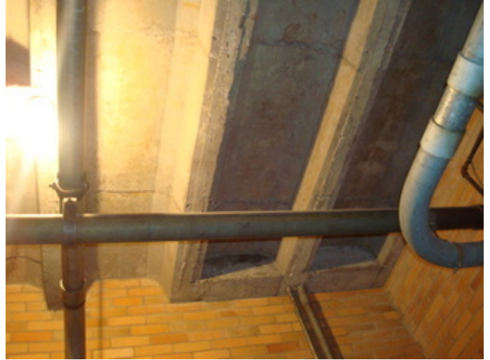
Underside of second floor
