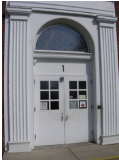
Typical hollow metal entry doors.
