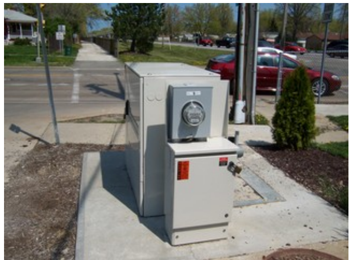
Pad Mounted Transformer
