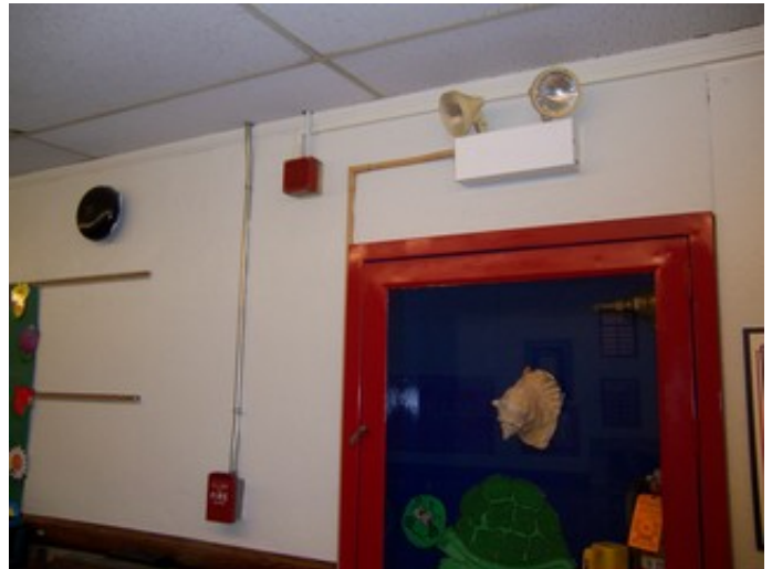
Typical Fire Alarm Devices
