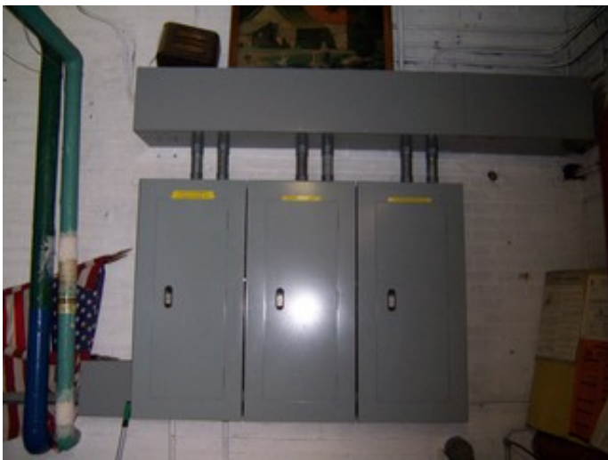
Electrical Distribution Panels 1, 2 and 3
