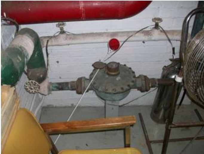
Domestic City Water Meter
