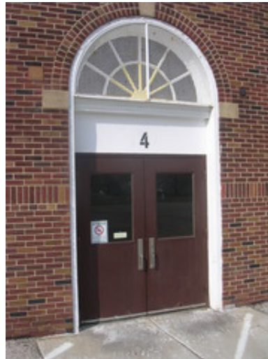
Typical hollow metal doors.
