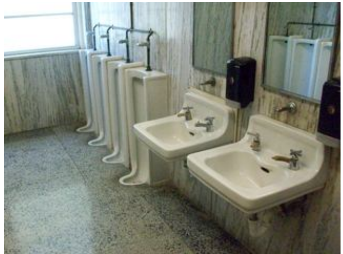
Typical Urinals and Sinks
