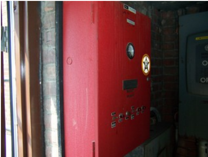
Fire Alarm Control Panel
