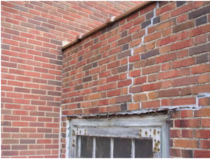
Failing window lintel and bulging masonry.
