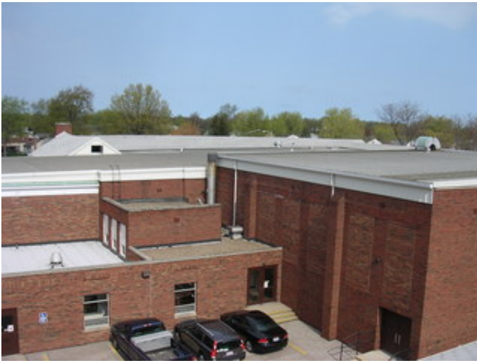
Typical roofing conditions.
