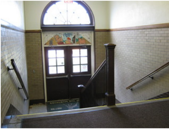
Steps at main entry
