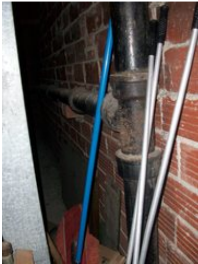
Sanitary Drainage Piping
