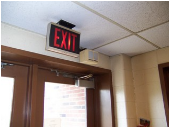
Typical Exit Sign
