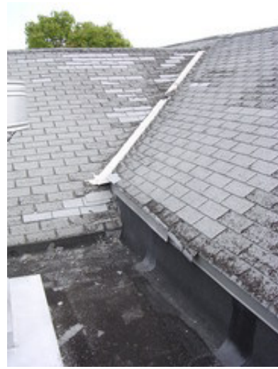
Asphalt shingles are in poor condition.
