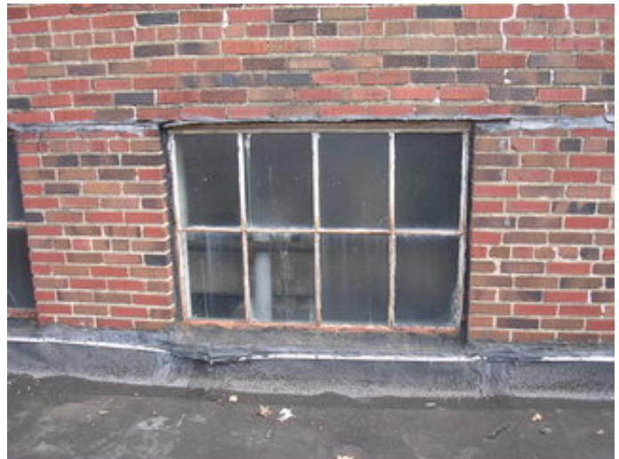
Steel frame window condition.
