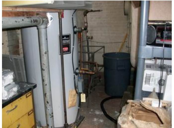
Domestic Hot Water Tank
