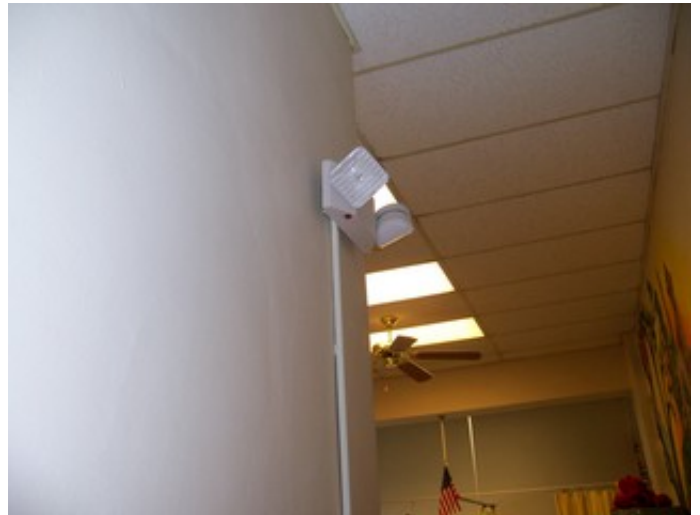
Typical Emergency Light
