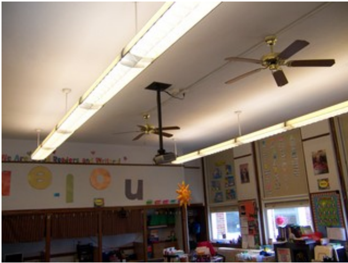
Typical Classroom Lighting
