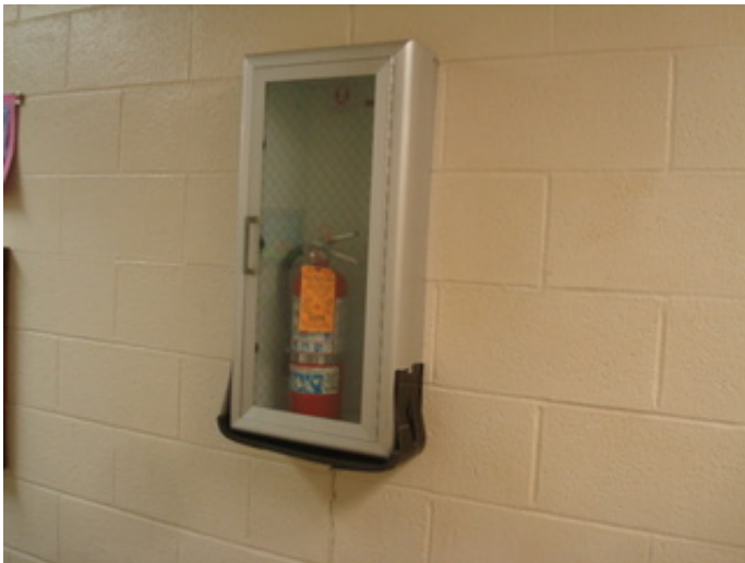
Fire extinguisher cabinet
