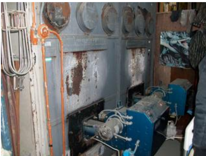
Gas Fired Hot Water Boiler
