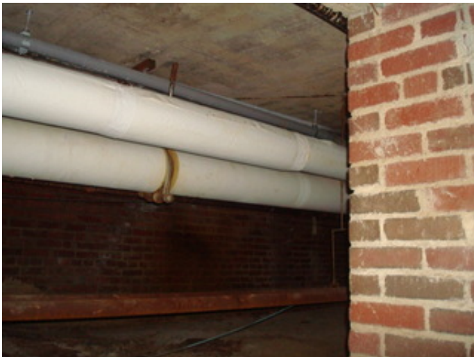
Pipes in tunnel
