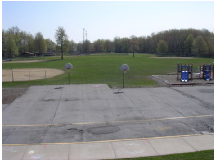
Playground and athletic facilities
