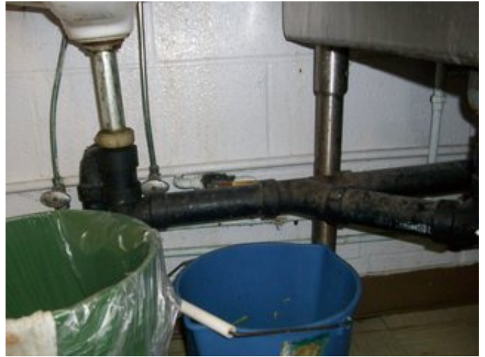
Sanitary drain below sink
