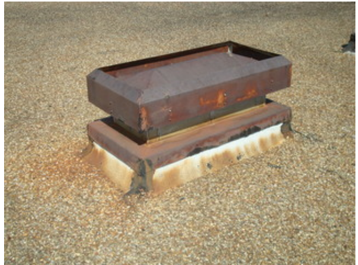
Hood with flashing that possibly leaks
