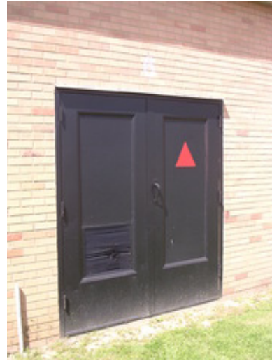
Typical hollow metal doors.
