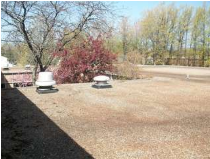
Exhaust Fans / Roof Ventilator
