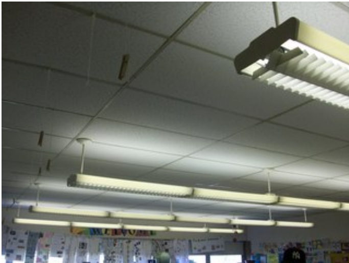
Typical Classroom Lighting
