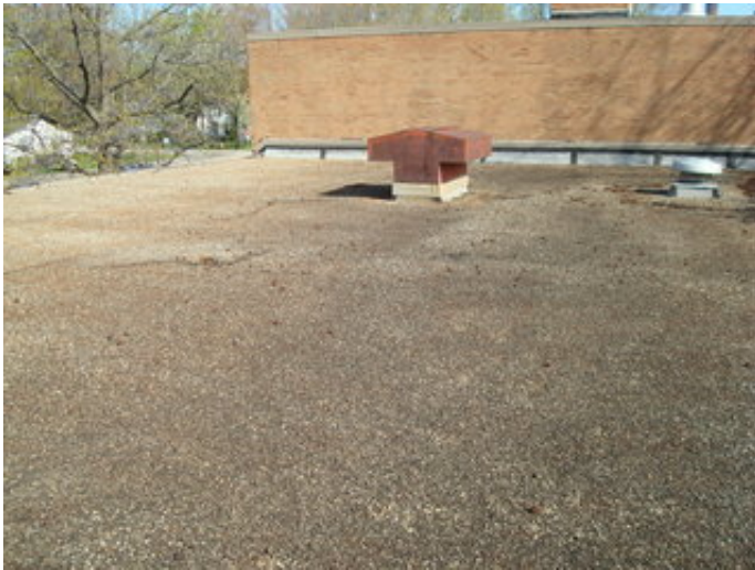
Evidence of ponding on roof
