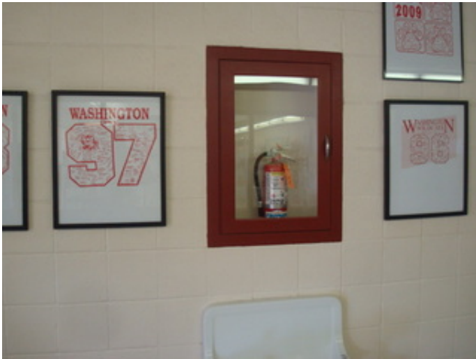
Fire extinguisher cabinet
