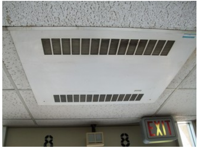
Ceiling Unit Heater
