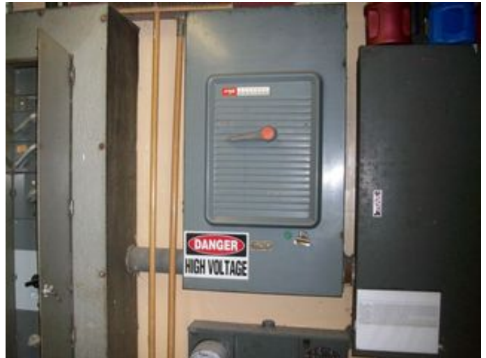
Main Electrical Switch Panel
