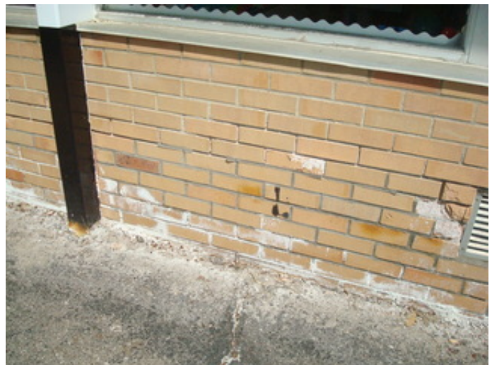
Damaged brick at South wall
