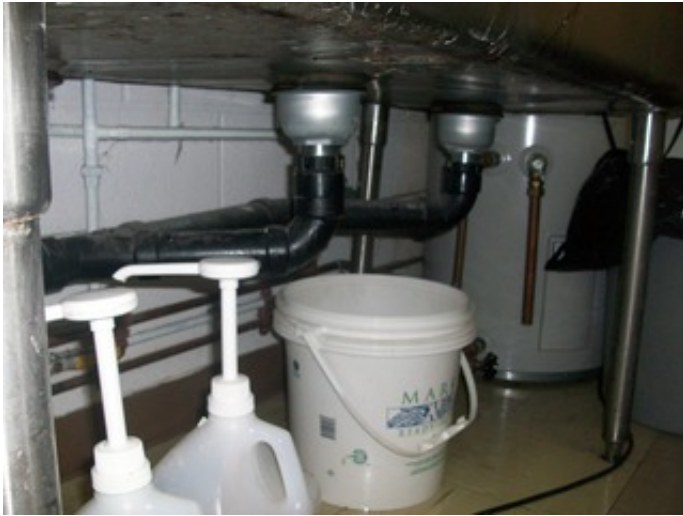
Sanitary drain below sink
