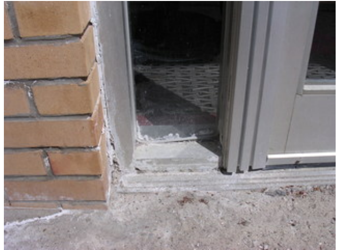
Aluminum storefront window system damage.
