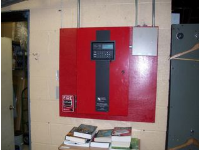
Main Fire Alarm Panel
