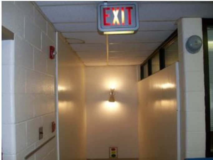
Typical Exit Sign
