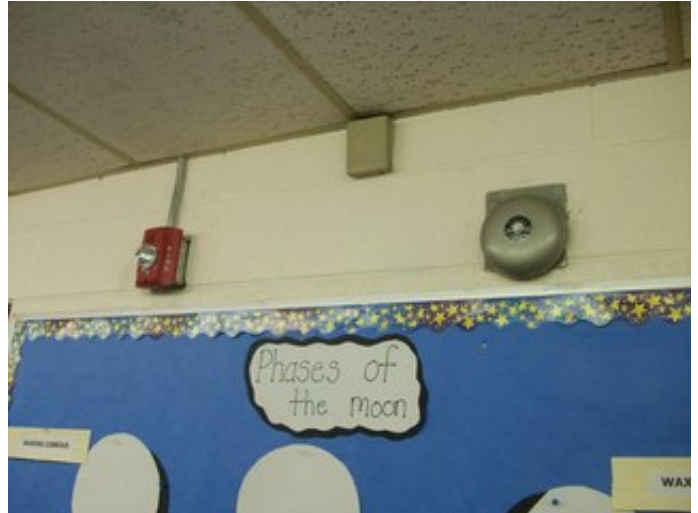
Typical Fire Alarm Devices
