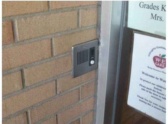
Main Entrance Visitor Intercom
