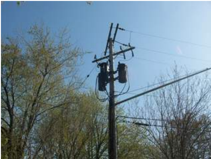
Pole Mounted Power Transformer
