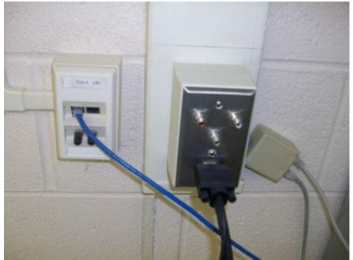
Typical Classroom Technology Port
