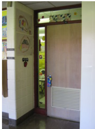
Typical recessed classroom door
