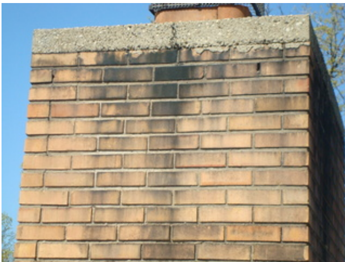
Damaged brick and coping at chimney
