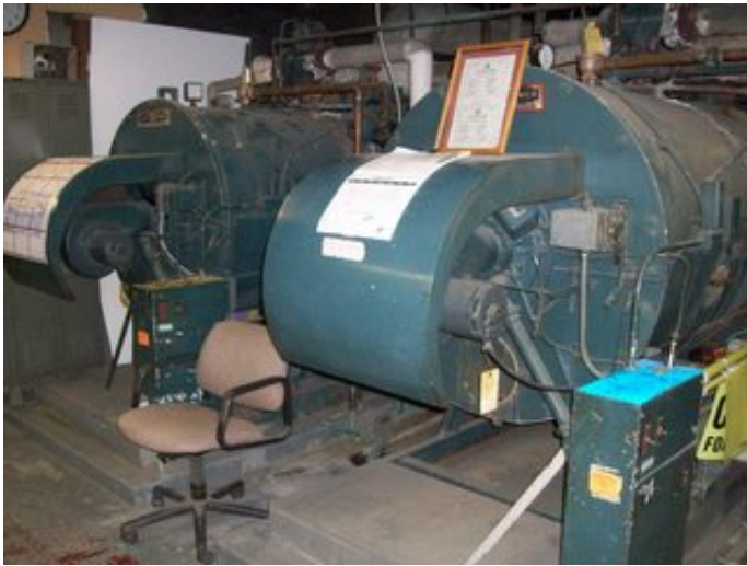
Gas Fired Hot Water Boilers
