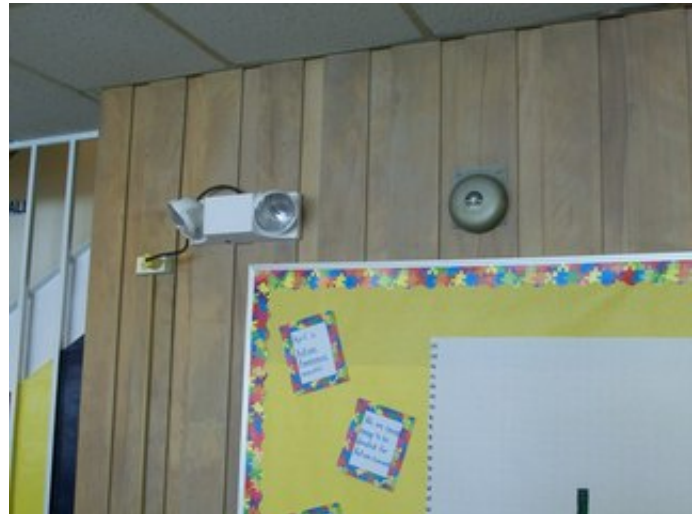
Typical Emergency Lighting Unit
