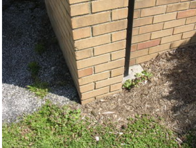
Typical foundation condition.
